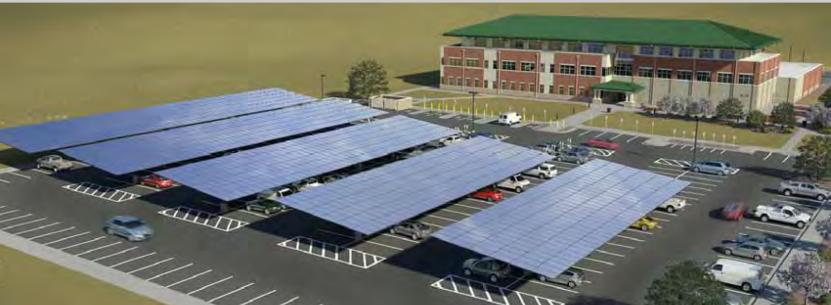
(ABOVE) A concentrated photovoltaic installation.
